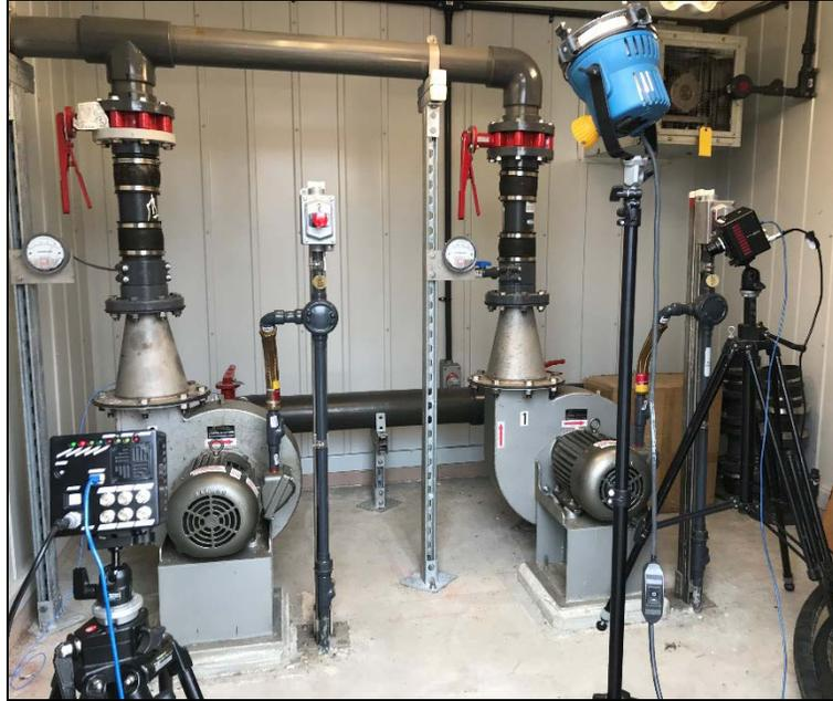
Figure 2: Picture of the example blowers, motors, and ducting, and their layout in the machine room.
